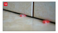
either with the load-bearing layers underneath or with the walls to its sides. Any unco-4 vered points that could constitute an "acoustic bridge" must be covered with Isolmant Fascia Nastro.
